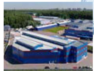
Stabilimento - Russia Plant - Russia
