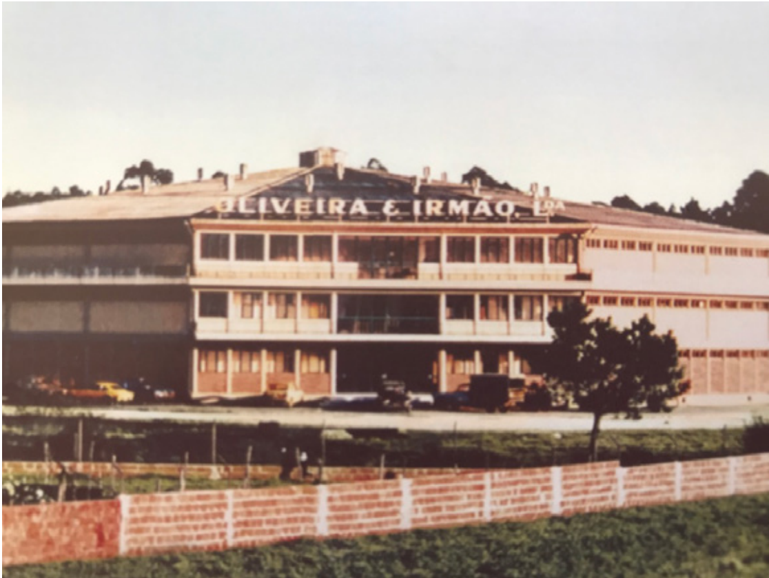
Company's headquarters in Esgueira
